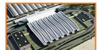
Expansion of Terminal 2
